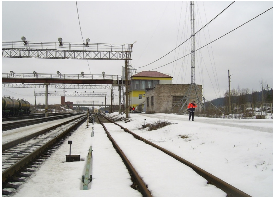
Figure 3.3.6.1 – Tracks No. 1 and No.10, light posts, inspection rams, antenna, service radio communication antenna, the old unused and the new building of RZD dispatch control service, paved area (view from the Russian side)
