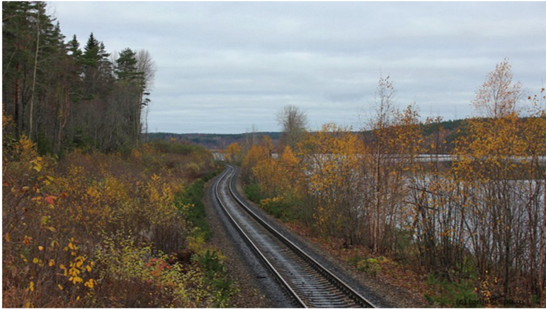
Figure 3.3.8.3 – Typical view of a section of the Kamennogorsk – Svetogorsk railway
