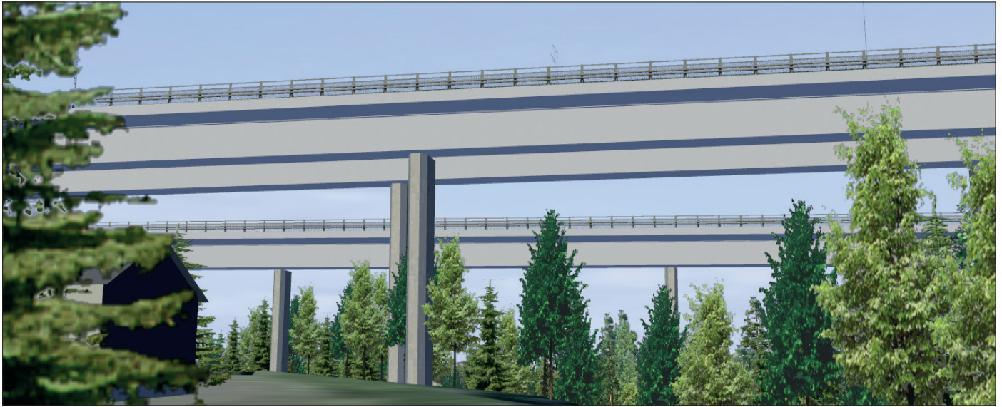
Demonstration of the new double track bridge over the Saimaa Canal. (Sito Oy)
